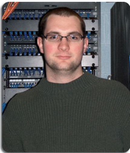
Josh Kolka, Technology Administrator for Bangor Township Schools, pictured here in one of the server rooms that he manages.
